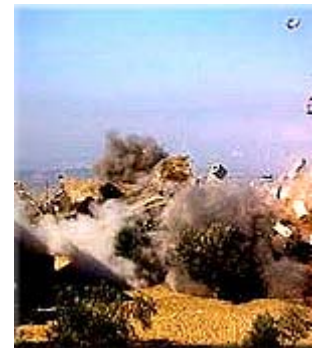
January 19 2003: Destruction of a house in Rafah by the IDF. No reason is given and the attack happened without warning the family in advance. The Palestinians have few rights under occupation. PHOTO: MOHAMMED OF RAFAH
